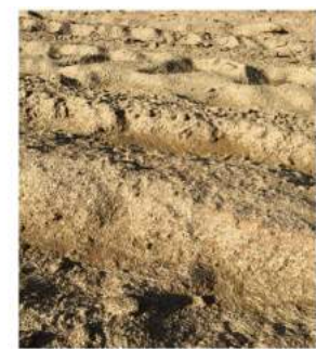
↑ Sloped areas were hydromulched at various stages and showed signs of water pooling
