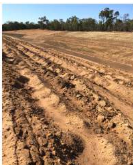
↑ A seedbed was prepared by ripping the sloped areas.
