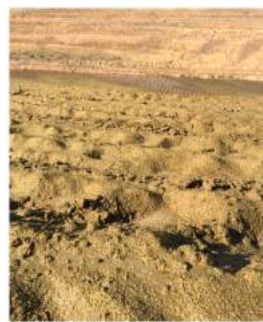
↑ Sloped areas were hydromulched at various stages and showed signs of water pooling
