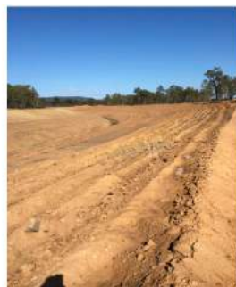
↑ A seedbed was prepared by ripping the sloped areas.
