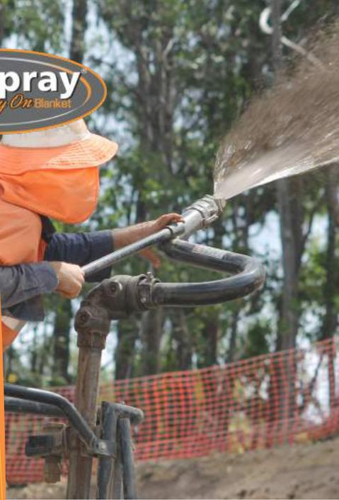
GeoSpray is applied with standard hydromulching equipment.
